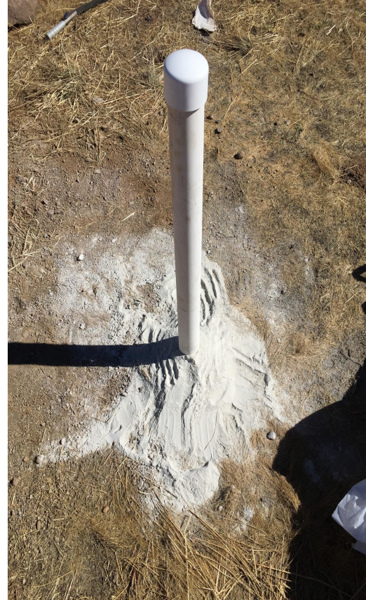
Figure 8: Packing monitoring well
